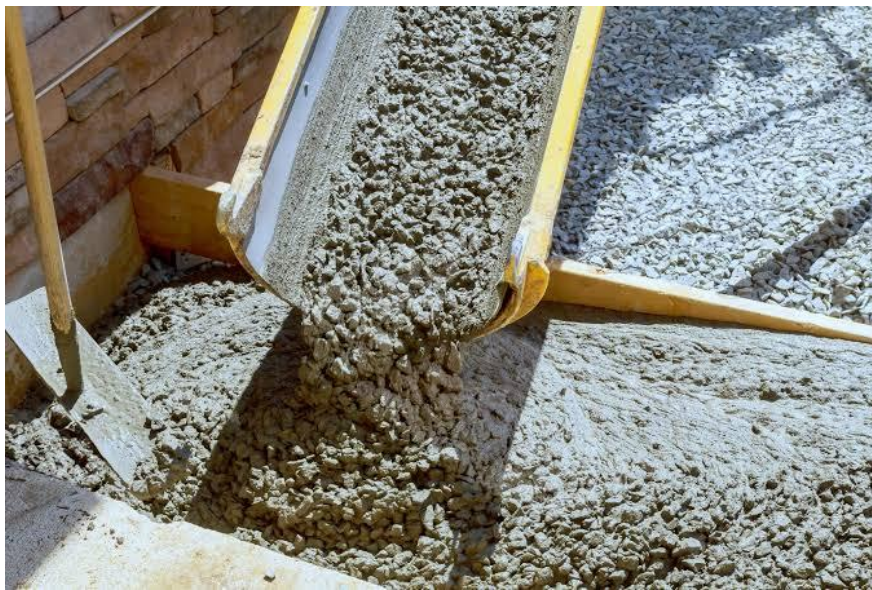
Figure 1: Concrete mixing and placement during the preparation of cementitious specimens.
