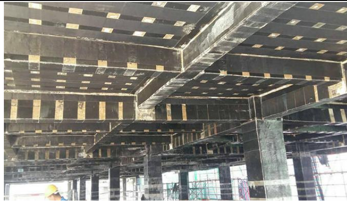
Figure 3: Fiber Reinforced Polymer
