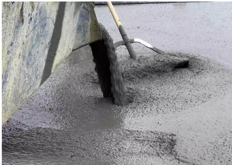
Figure 2: Self-Compacting Concrete (SCC) [6]
